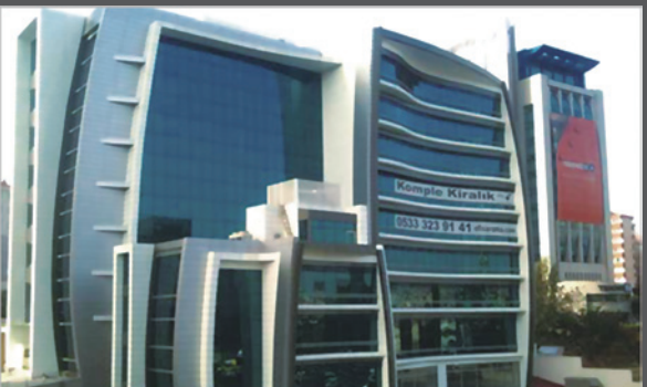
Office building in Istanbul,Turkey.
