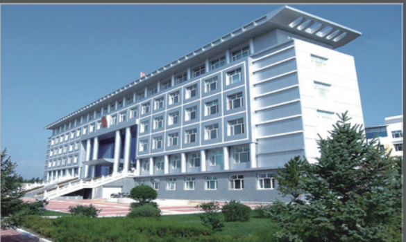
Government building in Inner Mongolia, China.
